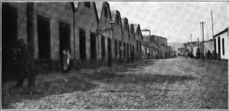
Street in Tacna Showing Earthquake Proof Houses
